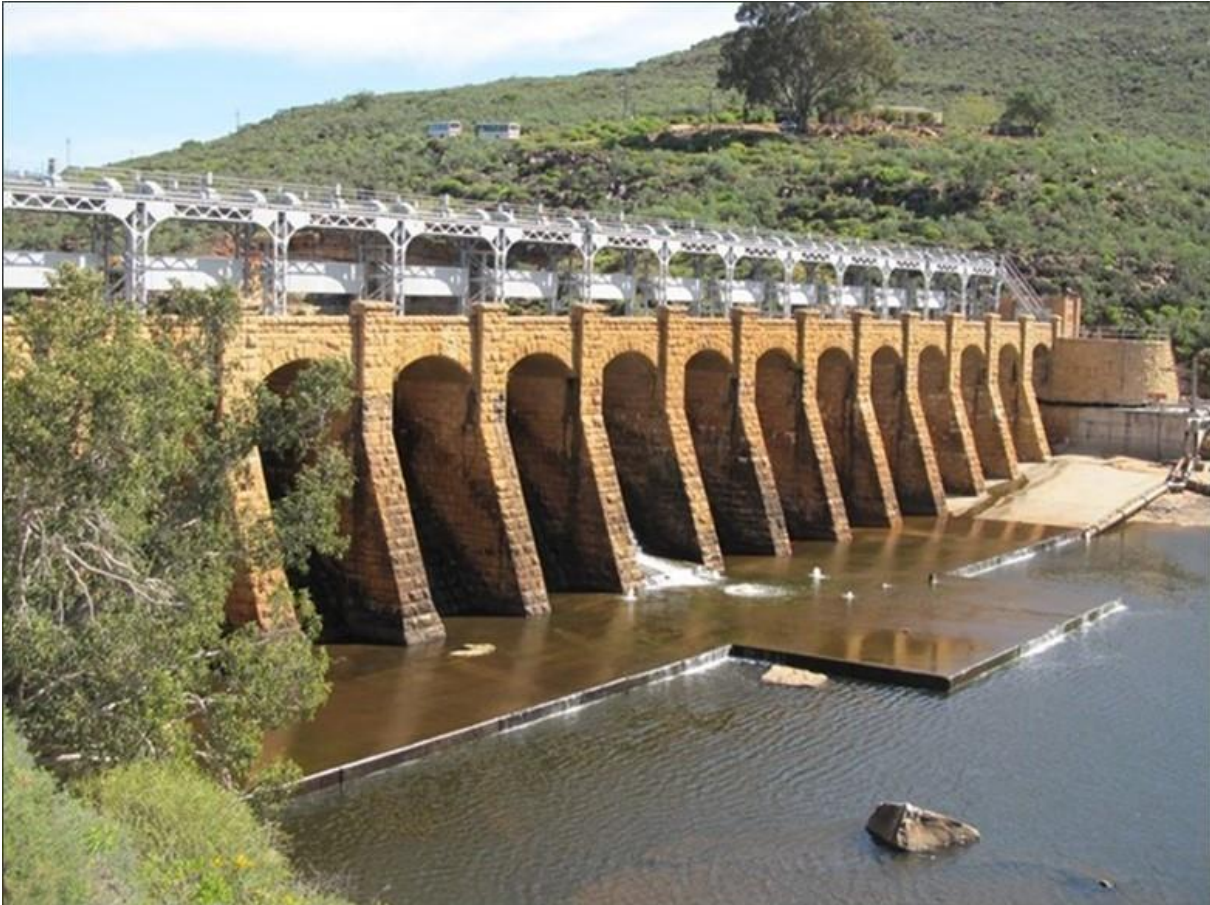
Figure 5.4: Concrete masonry Bulshoek Weir
