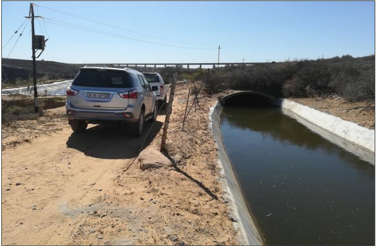
Figure 6.8: Abstraction point from the Retshof canal section
