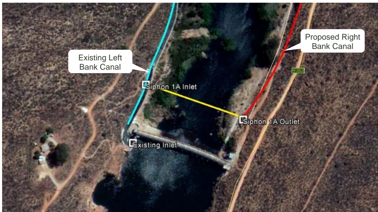
Figure 5.12: Syphon S1A at Bulshoek Weir
