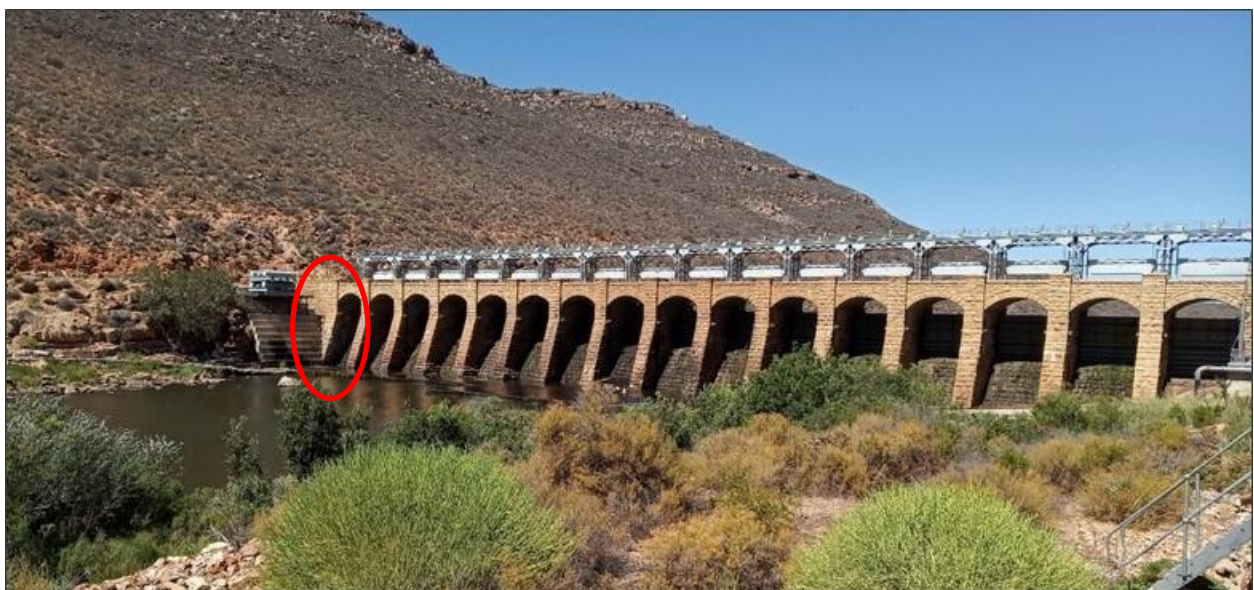
Figure 5.6: Last buttress gate at the Bulshoek Weir no longer in use
