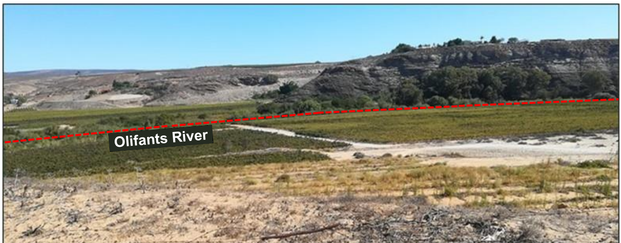
Figure 6.9: View from Retshof canal abstraction point towards Vredendal canal
